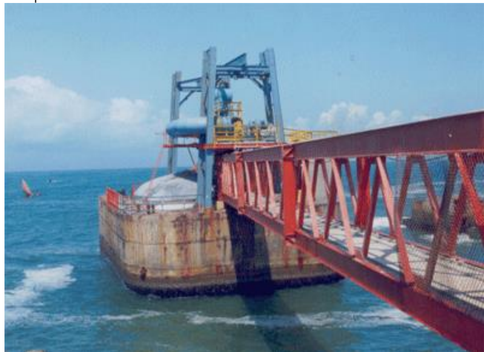
The Indian wave power pilot plant of 150 kW capacity in Arabian Sea
